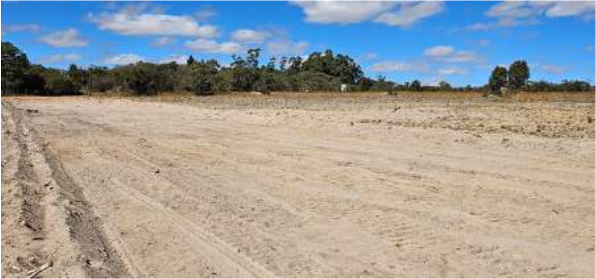
On going road construction in Elmswood residential area
