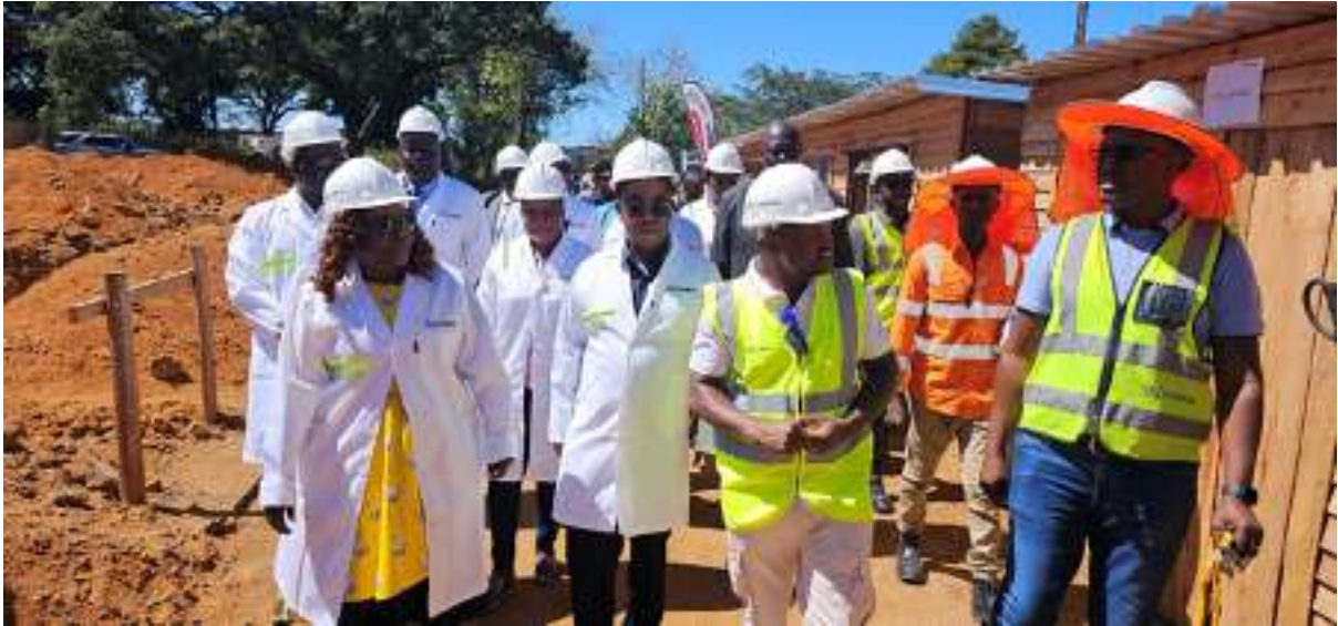
The Honourable Minister of State for Provincial Affairs and Devolution for Mash East, Hon. Dr. A Munzverengwi (Sen.) tours the NAC Headquarters construction site during the ground breaking ceremony while being guided by the site foreman
