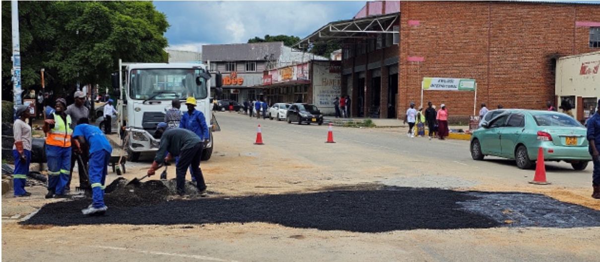
Re-tarring of a road section along second street
