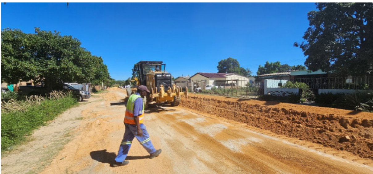
Dimba road resurfacing in Rujeko suburb
