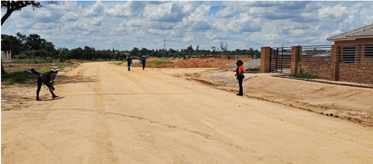
Council employees prepare a Ruzawi West Road for tarring
