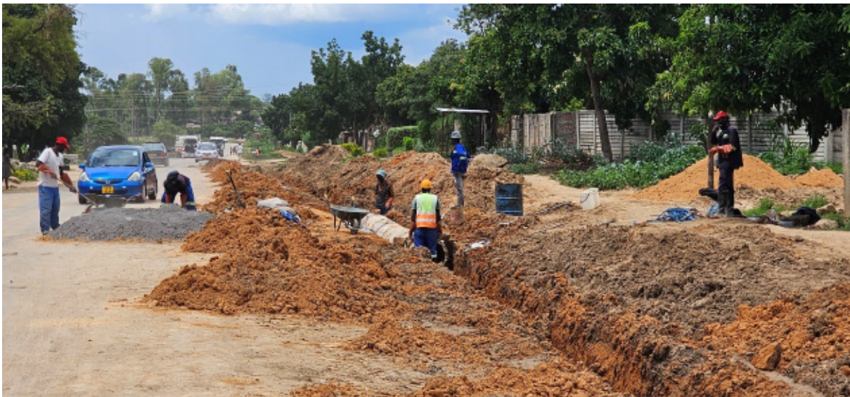
Council construction workers laying drains in Cherutombo residential area
