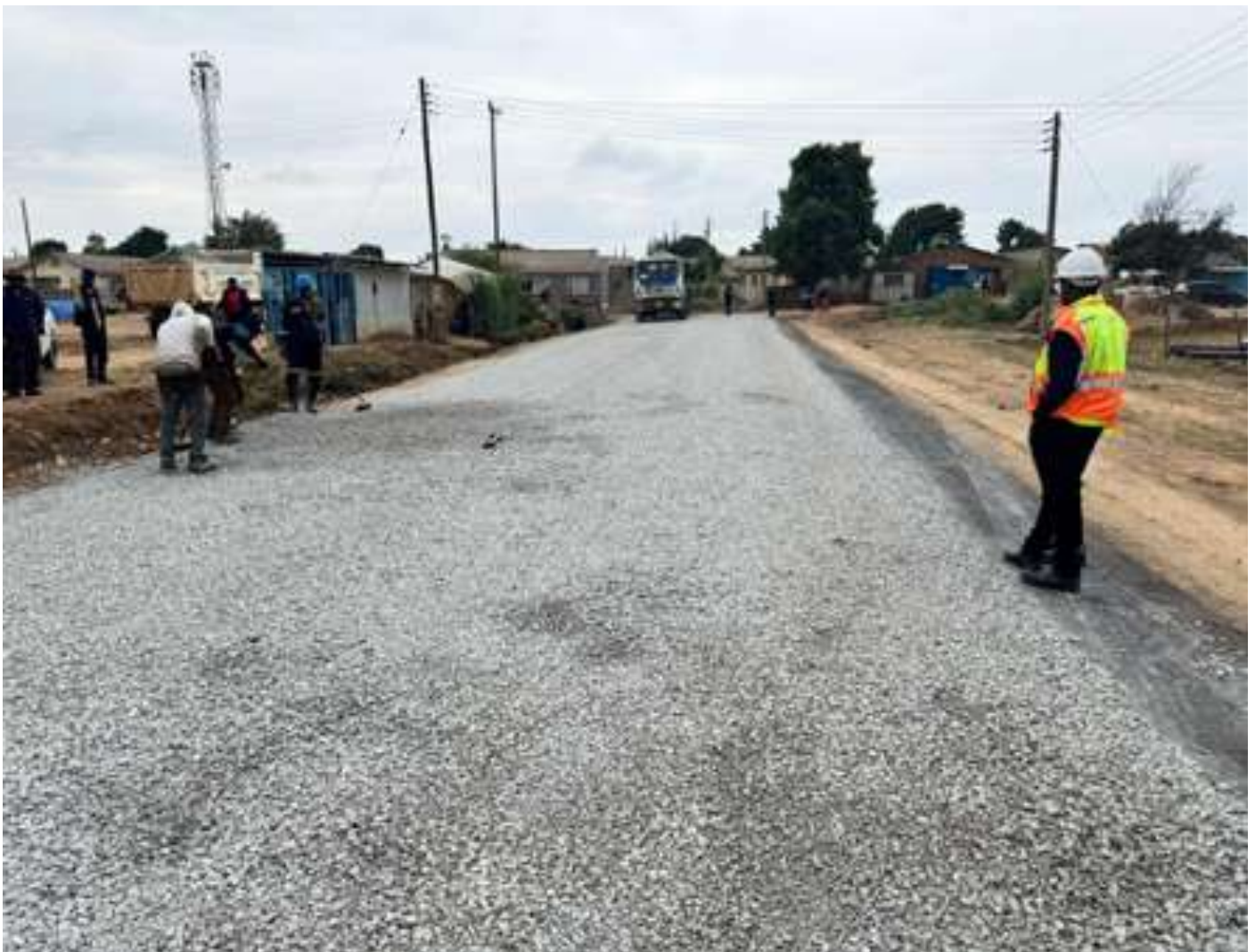
Mutufu Street Road works in Rusike Suburb
