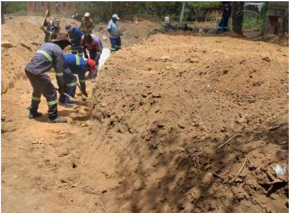
Council workers working on a drain
