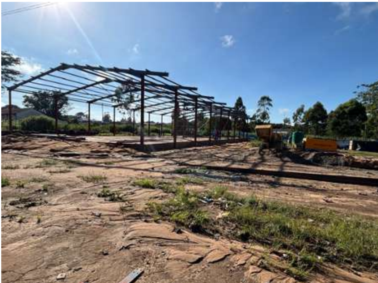
Construction works have commenced at the new 1st Street Market
