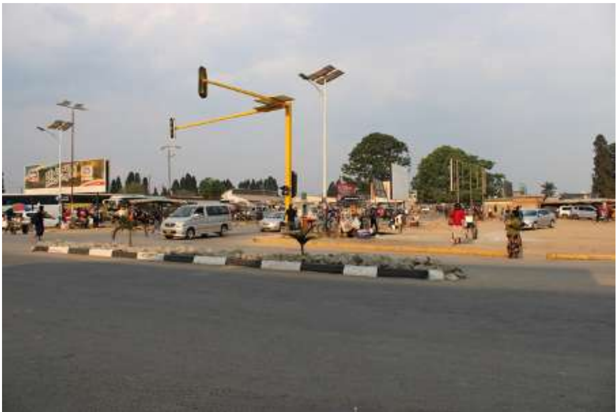
One of the new traffic lights installed at the corner of Pine Street and Ruzawi Road within the CBD to enhance traffic management
