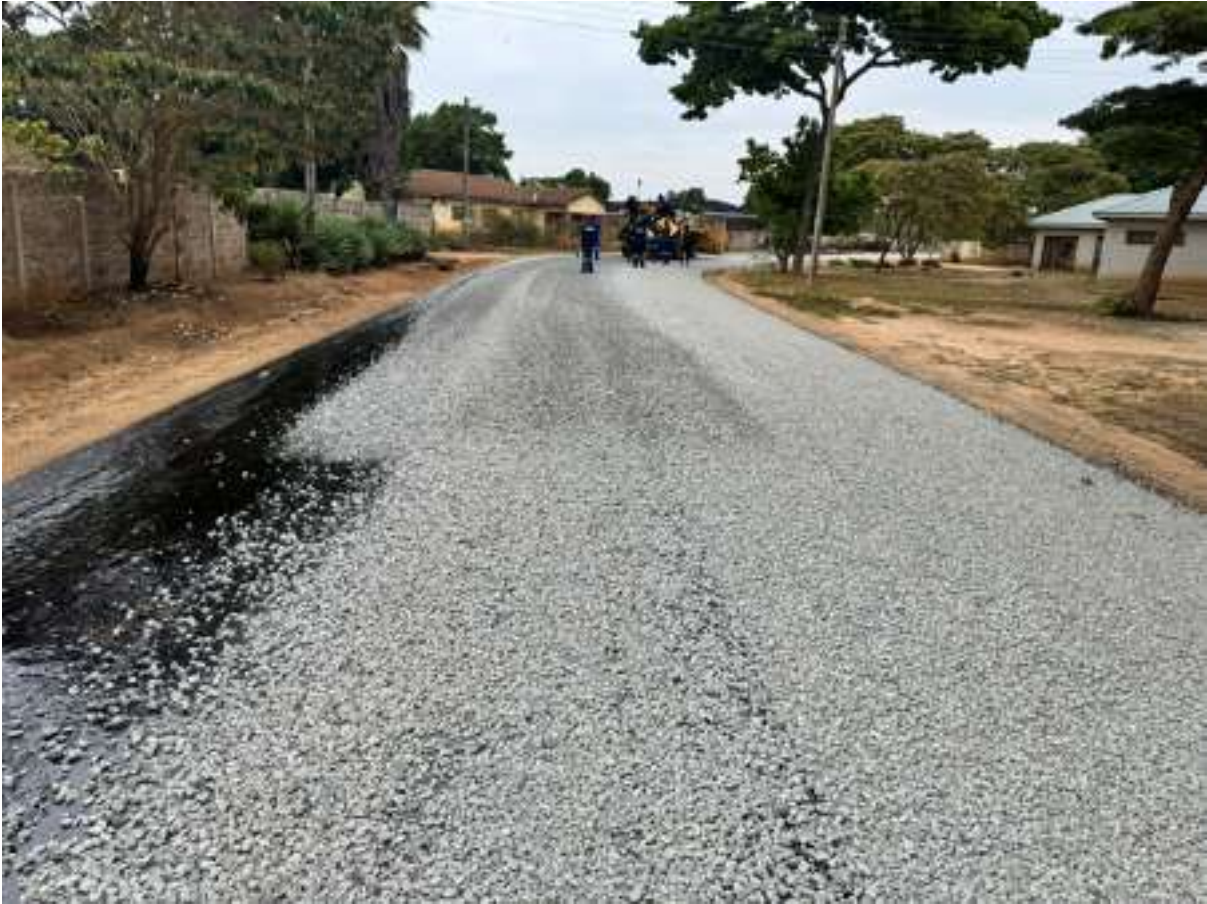
Mutiti road works in the Ruvimbo Park suburb
